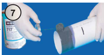
Solvent Cement Application
