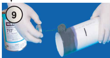
Solvent Cement Application
