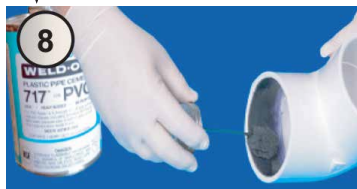
Solvent Cement Application
