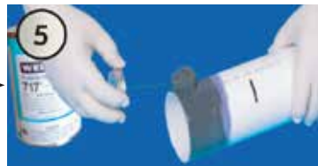
Solvent Cement Application
