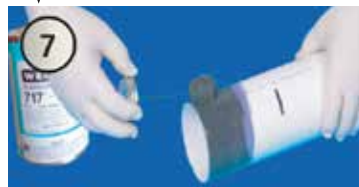
Solvent Cement Application
