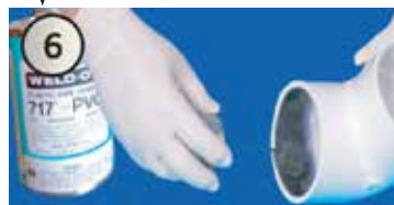
Solvent Cement Application
